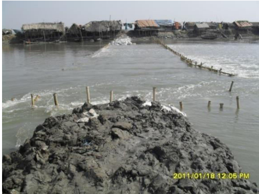
Courtesy: Bangladesh Water Development Board
