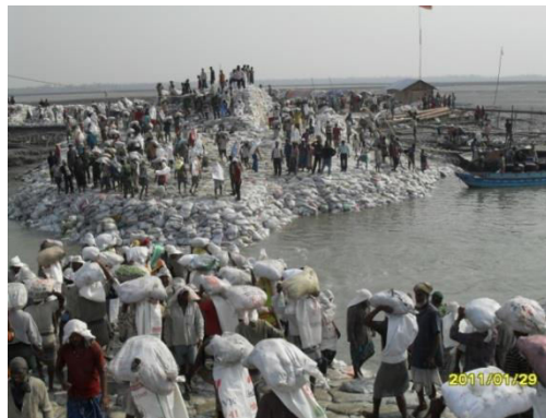
Courtesy: Bangladesh Water Development Board
