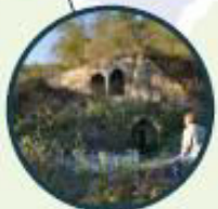
Crystal Wall Restoration project on St. Cuthberts Way
