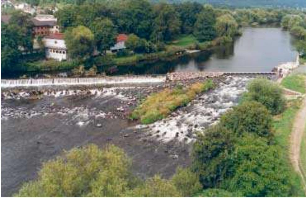
Figure 2. New designed weir with fish- ramp and control station for fish migration on the lower reach of the river Sieg
