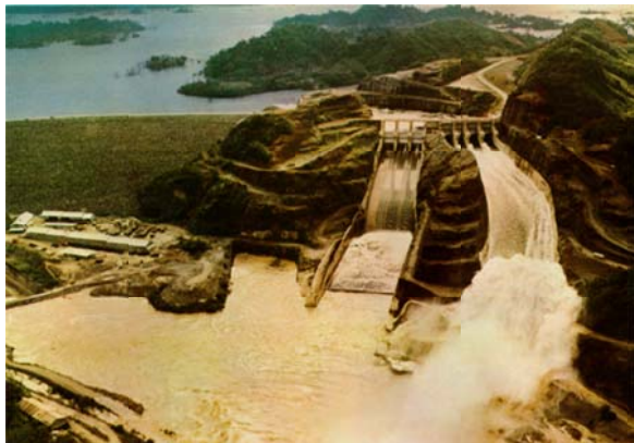
Figure 1. Operation of the emergency spillway (HRS, 1976)
