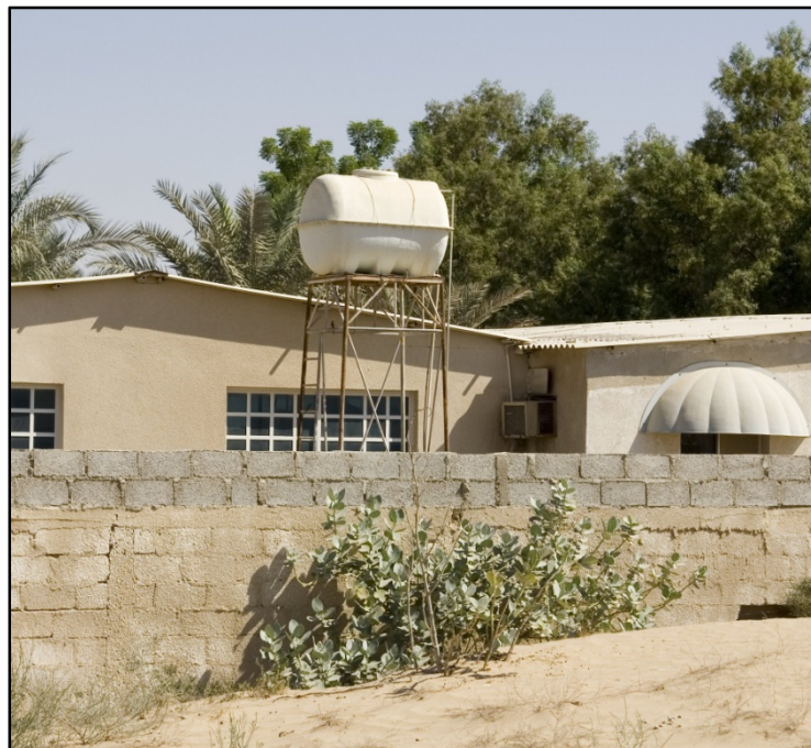
Figure 1 – Example of a user-serviced exterior water storage tank.
