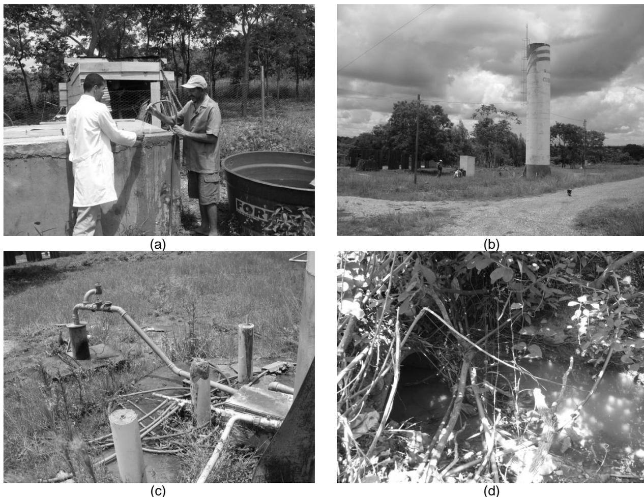
Figure 1. Community Cinturão Colina Verde, in Cuiabá city, Mato Grosso state: water collection in house (a); reservoir of the community (b); pipes of water distribution (c); water net in contact with wastewater (d)
